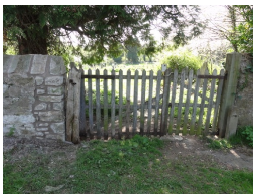
Wall repairs at the north gate.
